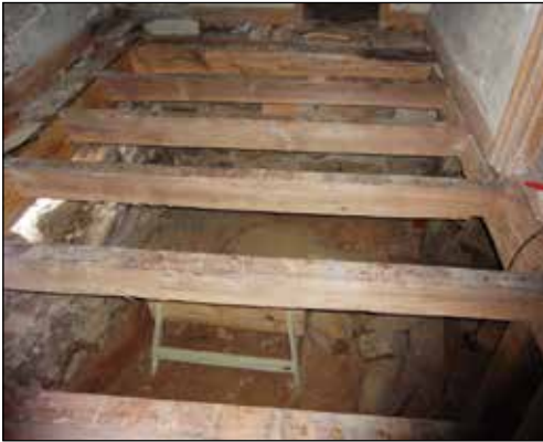
New floor joists were created to replace the ones destroyed by water damage and termites.
