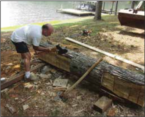
Tom King uses a broad axe to hew a new structural support beam for the floor at the Edward Dromgoole House in southern Virginia.
