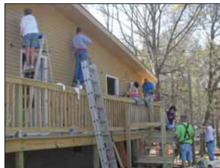
▲ A mission team from Main Street UMC in South Boston, Farmville District, traveled to Douglas County, Georgia, and worked on three homes that had been damaged by floods. Two weeks later a follow-up team returned and finished up so the families could return to their homes.
