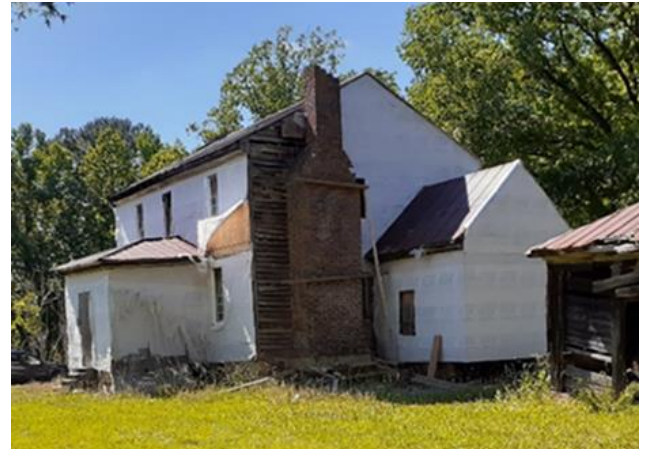
Dromgoole House -- east chimney braced after it began to tilt in 2019
