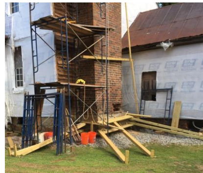
Braced East Chimney of Dromgoole House
