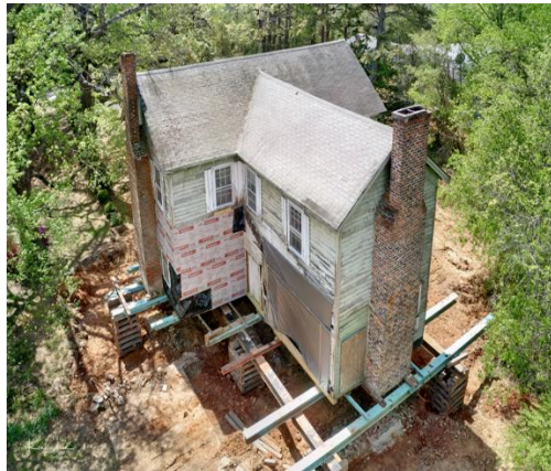
Aerial back view--Cottage raised off its original Foundation (Photo courtesy of Ken Currin)
