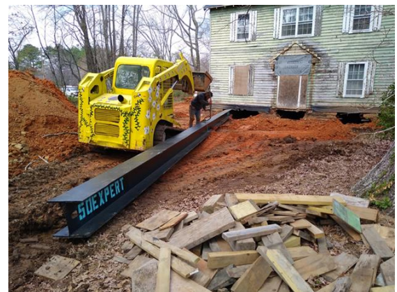
Metal beams being placed underneath
