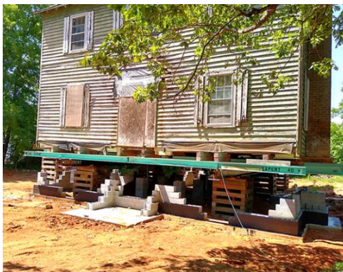
Concrete footing poured & new foundation built
