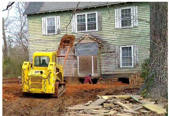
Excavating dirt from underneath the cottage
