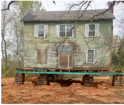
Front View--Cottage lifted off its original foundation
