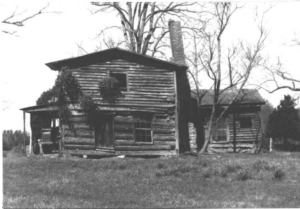
FIGURE 10 Main House, South Side of Route 58, .86 of a Mile East of Route 677
