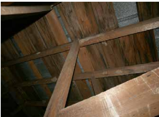
Attic, showing typical common rafters and sheathing (2022, left) and joists (Corker, right).
