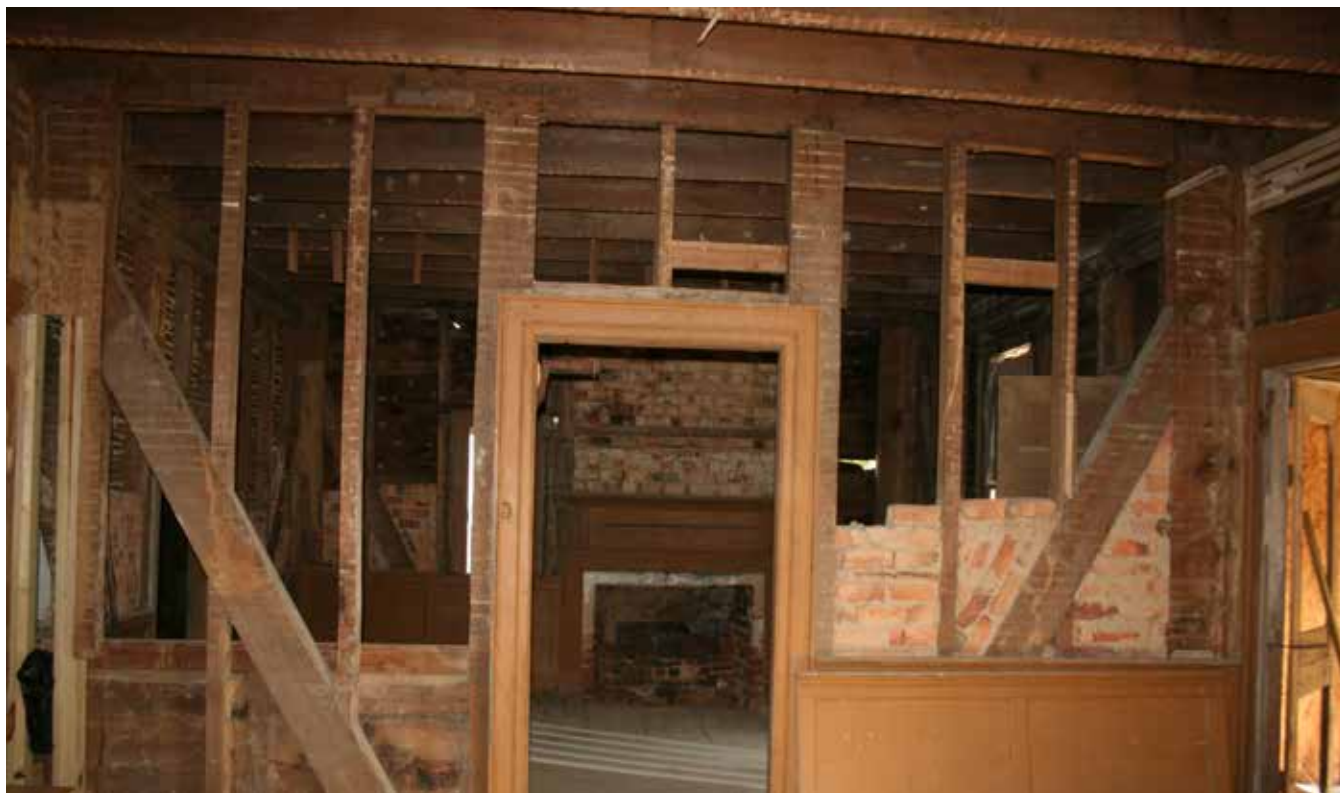
Hall looking east (above) and detail of central partition with intact brick nogging looking east (below), 2021.
