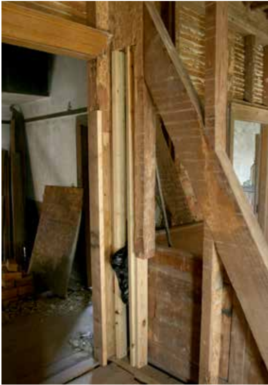
Rebuilt post at the north end of the first-floor partition between the Hall and the Parlor (left) and termite damage at the north end of a beam where it ends at the replaced sill under the north wall (right).
