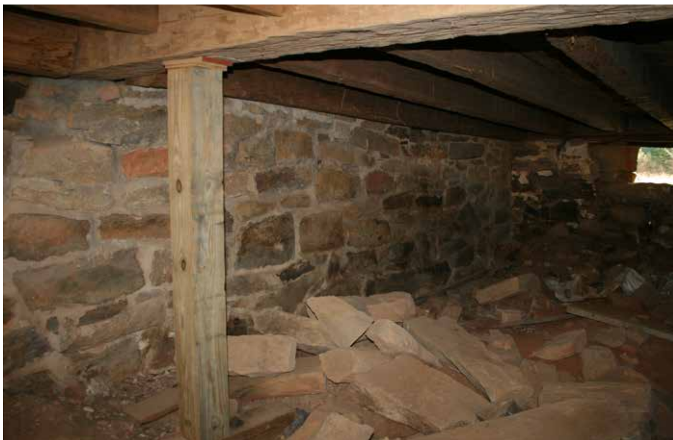
Basement, original stone pier looking southwest (above) and eastern room looking southeast at rebuilt stone wall (below), 2021.
