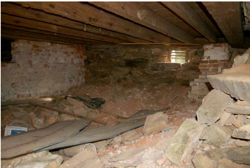
Basement, West Room, looking southeast showing central brick cross partition (left). Added brick bulkhead on the right.
