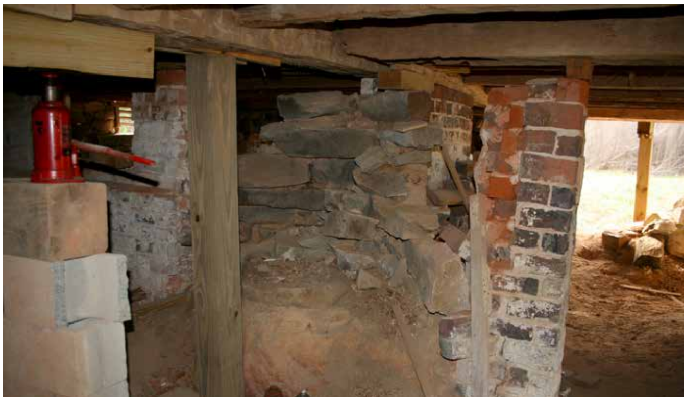
Basement, original stone pier looking southwest (above) and eastern room looking southeast at rebuilt stone wall (below), 2021.
