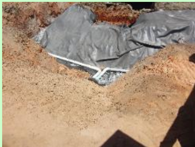
Drainage pipes with holes changes to solid pipes when it turns to go down the hill
