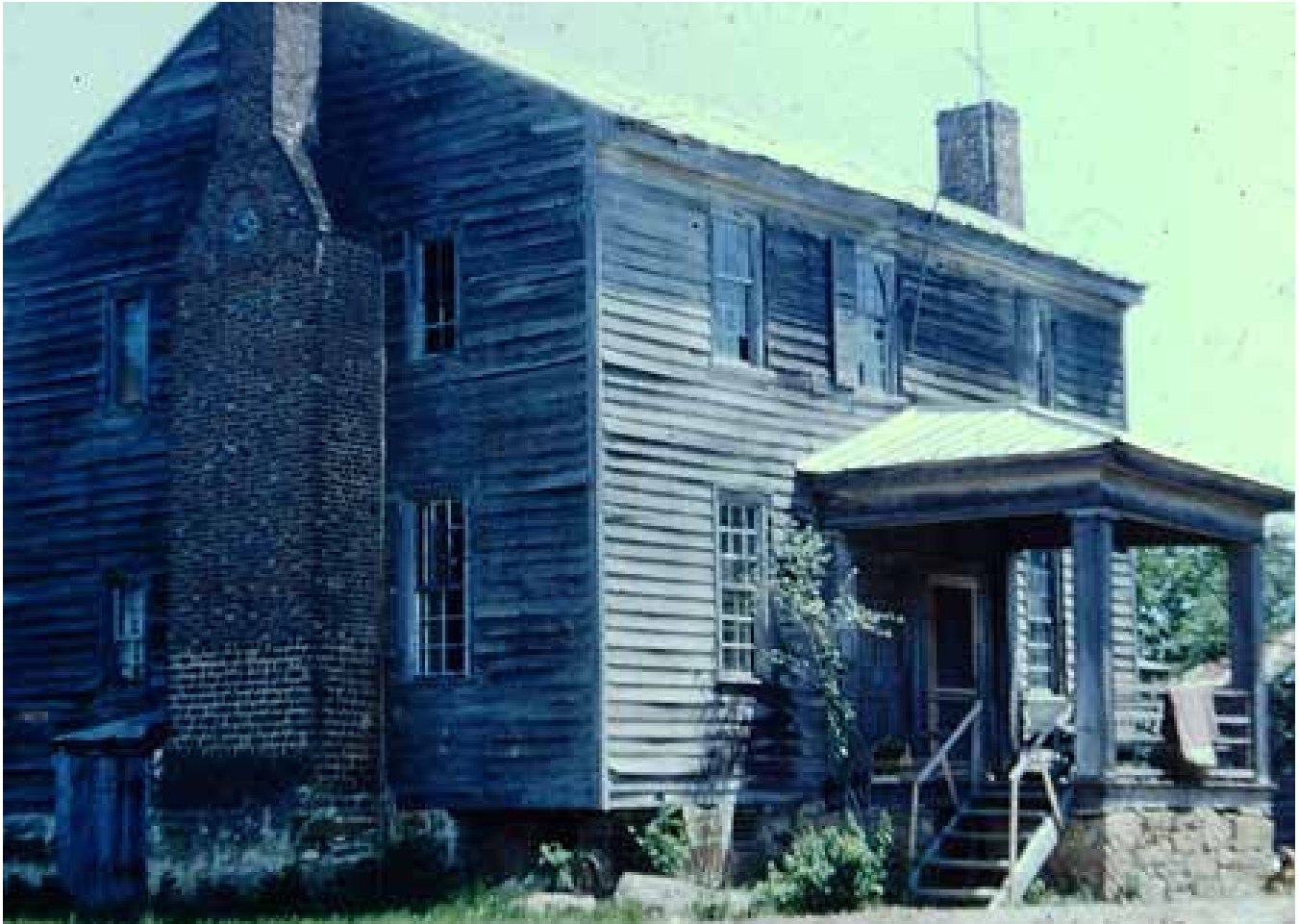
Southwest corner from southwest showing missing section of foundation, 1960s. A earlier basement entry is visible beside the chimney [Collection Old Brunswick Circuit Foundation].
