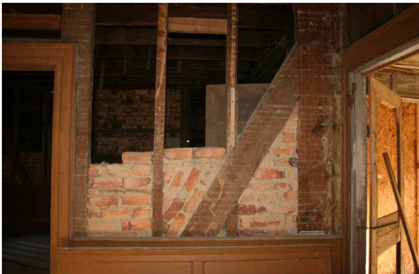
Hall looking east (above) and detail of central partition with intact brick nogging looking east (below), 2021.
