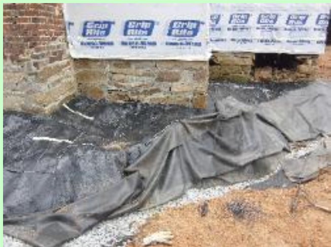
Voltex DS before the no. 3 stone with the pond liner not placed completely over it yet. The pond liner does not have a shiny surface, but the Voltex DS top layer is shiny.
