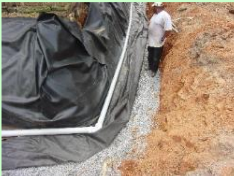
Above: Pipe on Geotextile filter fabric, with Voltex DS and pond Liner on the slope.
