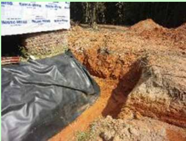
Pond liner – the trench out to the lower right in this photo is the one connecting to the Spinning House trench.
