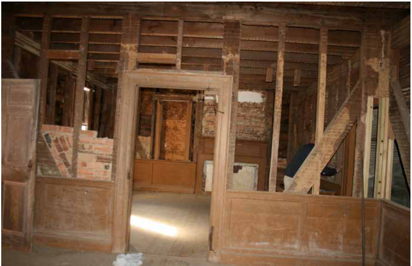
Parlor, detail showing framing and pegs attaching porch pilasters to frame looking south (above) and Parlor looking west (below), 2021.
