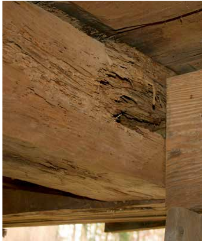
Rebuilt post at the north end of the first-floor partition between the Hall and the Parlor (left) and termite damage at the north end of a beam where it ends at the replaced sill under the north wall (right).
