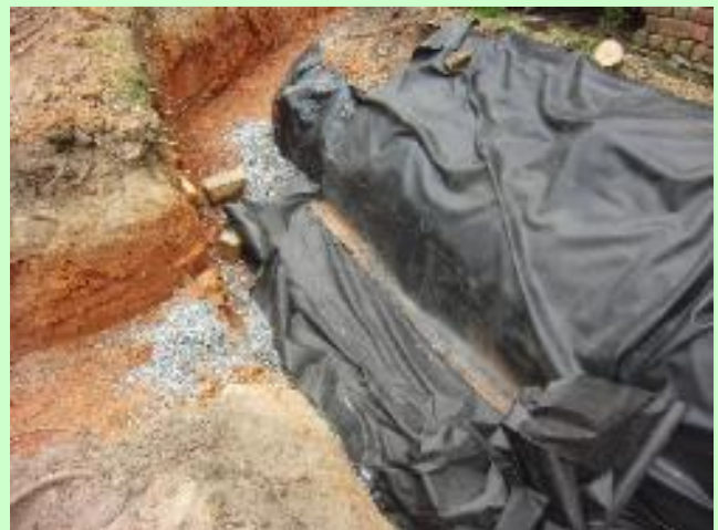
Geotextile Filter fabric at the bottom of the trench, Voltex Ds and Pond Liner on the slopes
