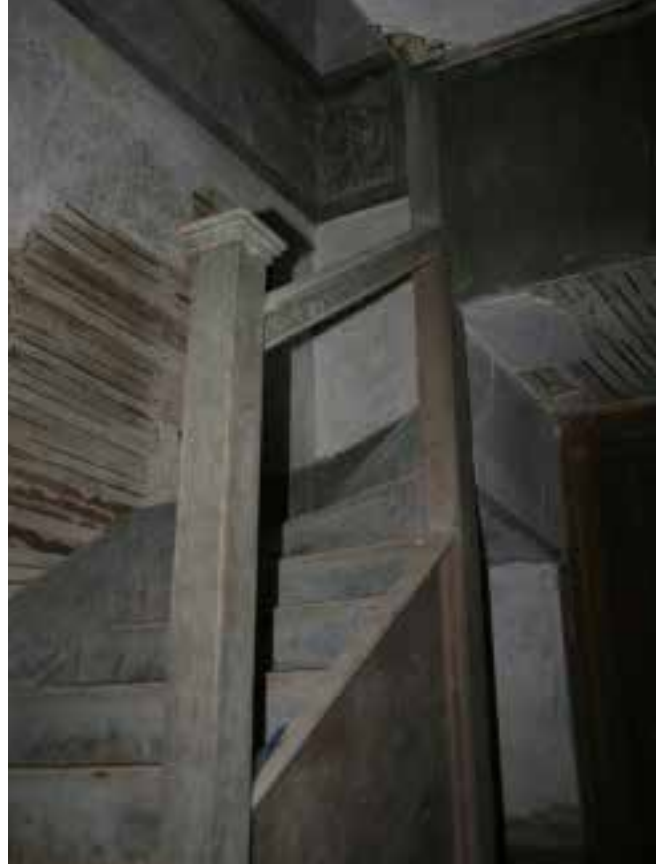
Decorative painting and graining at closet door under stair (left) and stair rail with missing balusters (right).
