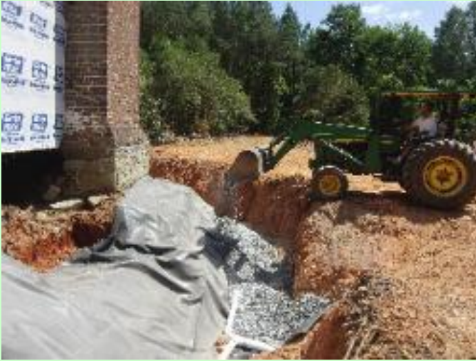
Top no. 3 Stone covering the pipe which drains down the hill starting on the northwest corner of the house.
