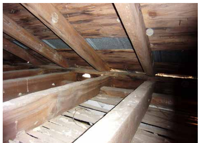
Attic, showing typical common rafters and sheathing (2022, left) and joists (Corker, right).
