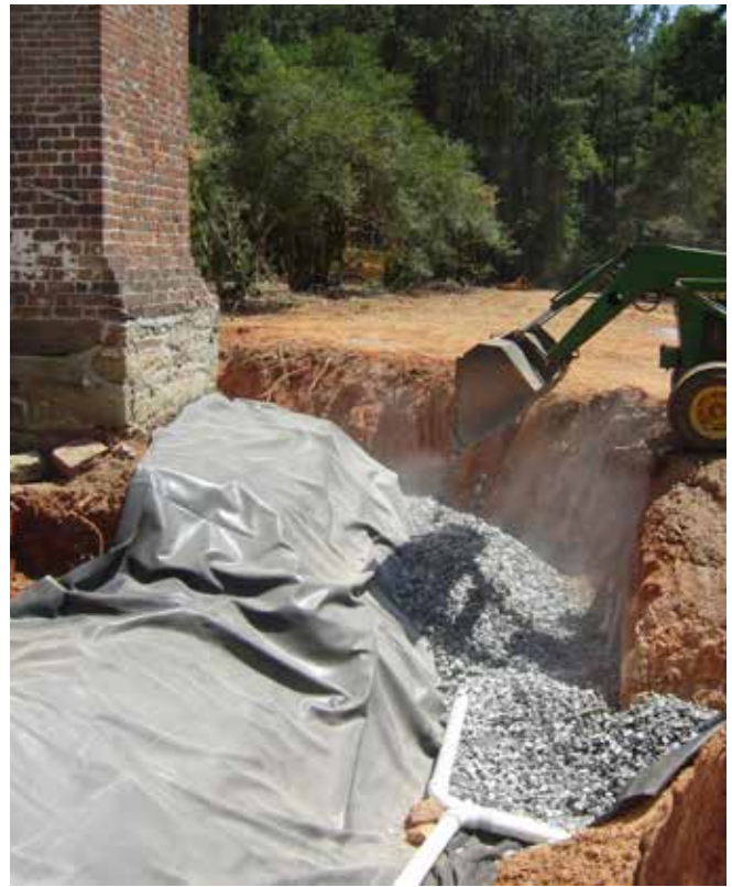
East chimney base during repair in 2013 (left) and west chimney during foundation drain installation (right).
