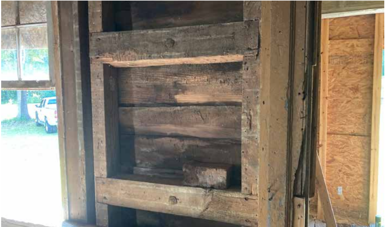
Parlor, detail showing framing and pegs attaching porch pilasters to frame looking south (above) and Parlor looking west (below), 2021.
