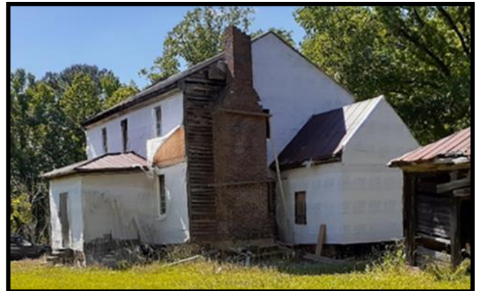
Right: Covered in a protective wrap in 2009, Chimney braced in 2019
